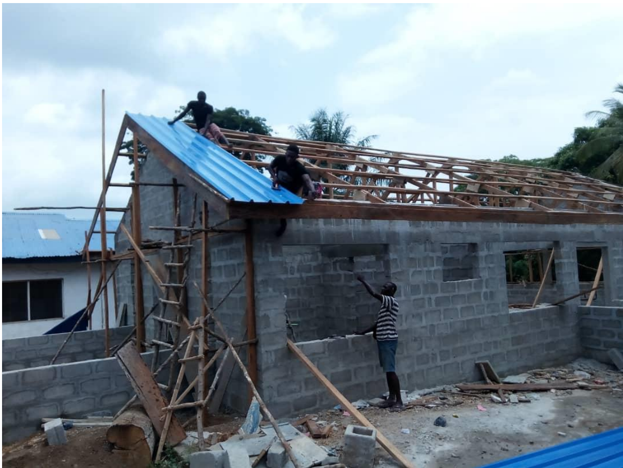
Total renovering af maternity ward
